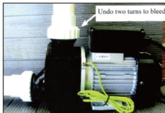
If initial non starting or error messages HL, LF, dr & dy, these error warnings normally indicate "air lock". Do as below to release "air lock": turning off the power supply, undoing the highest pump coupling on the circ pump two turns by a large wrench, until you hear air escape(some water also escapes), and gently shaking the pipe or hose attached to the pump until any air pocket has escaped from the pump. Retighten the pump collar and repeat start up procedure.
